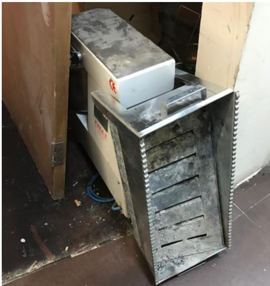
sf015 - Ground Floor corridor – Burner Photograph taken on 13 June 2019 @ 11.59hrs
